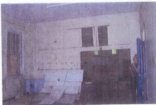
Timber dividing walls
